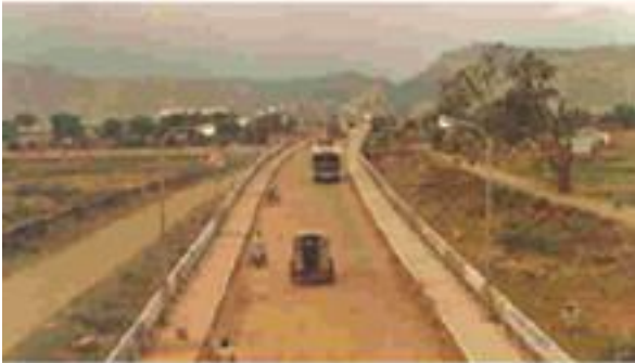
Road over-bridge Alwar
