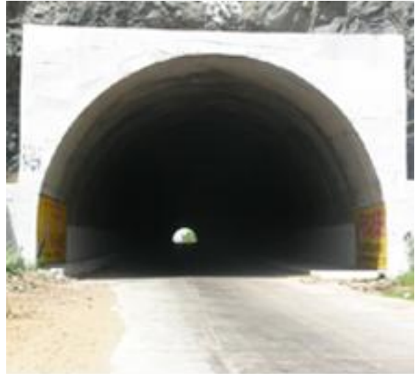
Jindoli Bypass Tunnel Alwar
