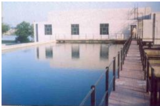
Photo 4.2 View of water filtration plant
