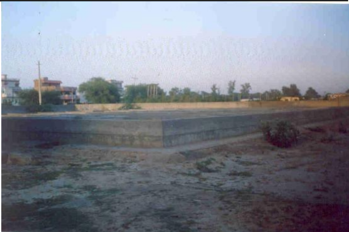
Photo 4.4 View of underground water tank under construction
