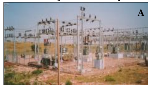
Photo 4.16 Projects funded by NCRPB
