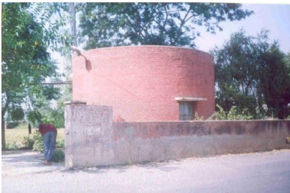
Photo 4.10 View of existing sewage pumping station (SPS)
