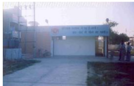
Photo 4.3 View of underground water tank with booster station
