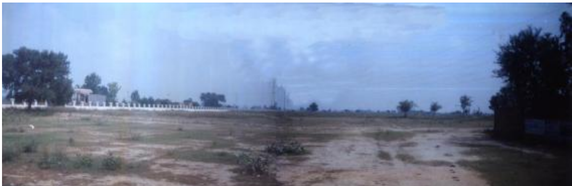
Photo 4.8 Site photograph of proposed Integrated Township at Baran showing boundary wall constructed
